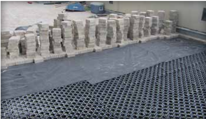
Figure 7. Concrete pavers on geotextile over plastic grids
